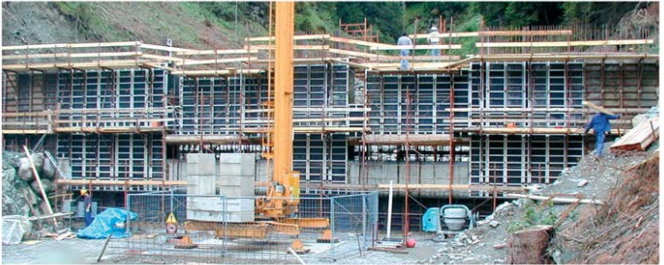
Dam WALL with COM PANE Alu (AUSTRIA)
