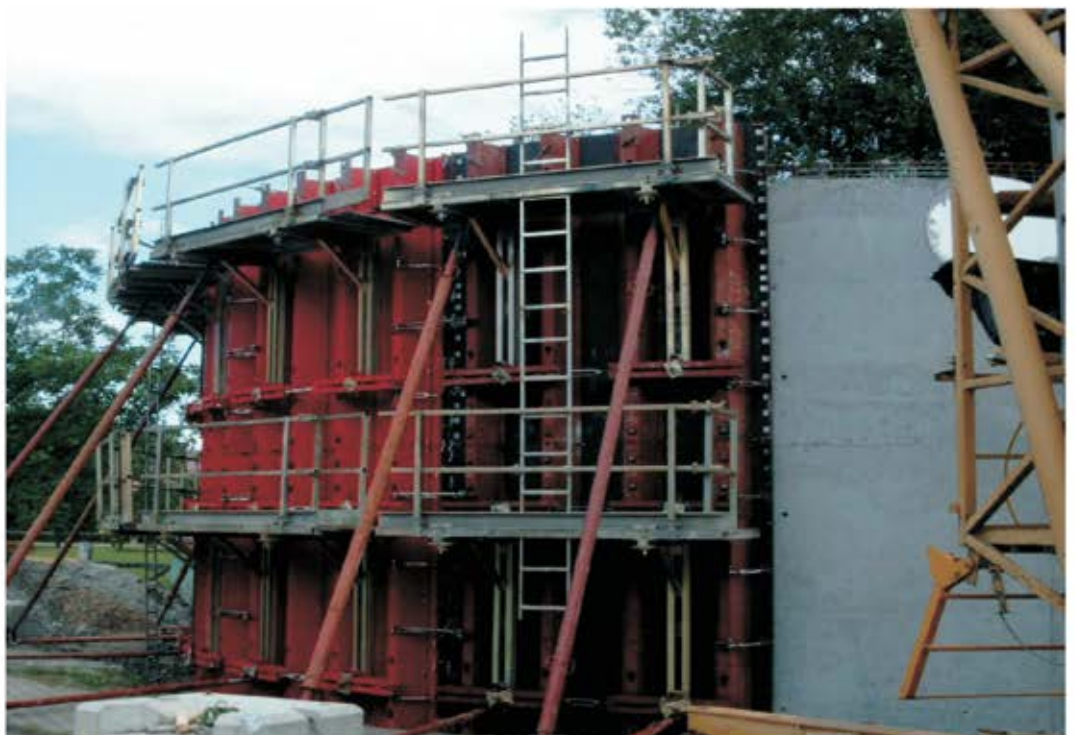
SHOWING FORM & CONCRETE FINISH
