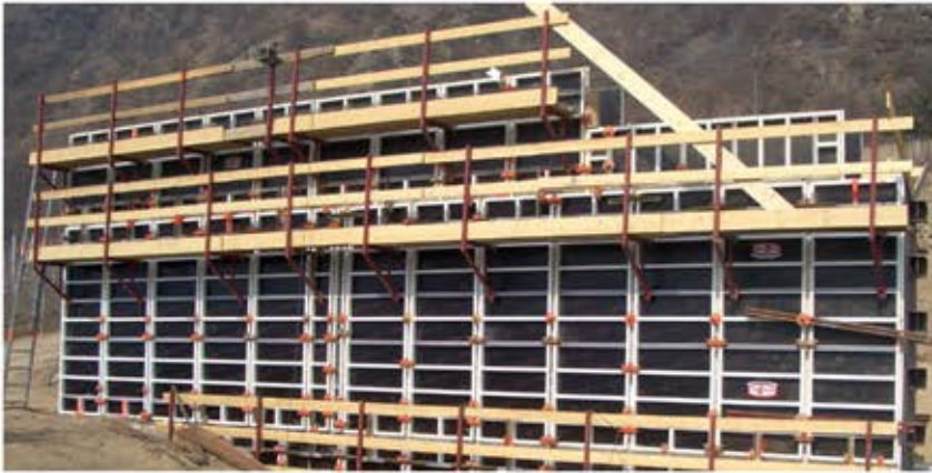
COM PANE Alu formwork, 7 m high
